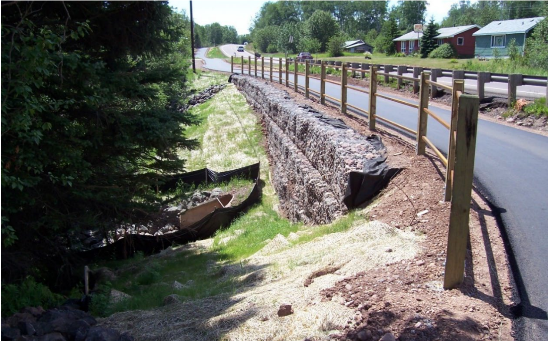
This image shows vegetative coverage of around 50%v and would not be acceptable.
