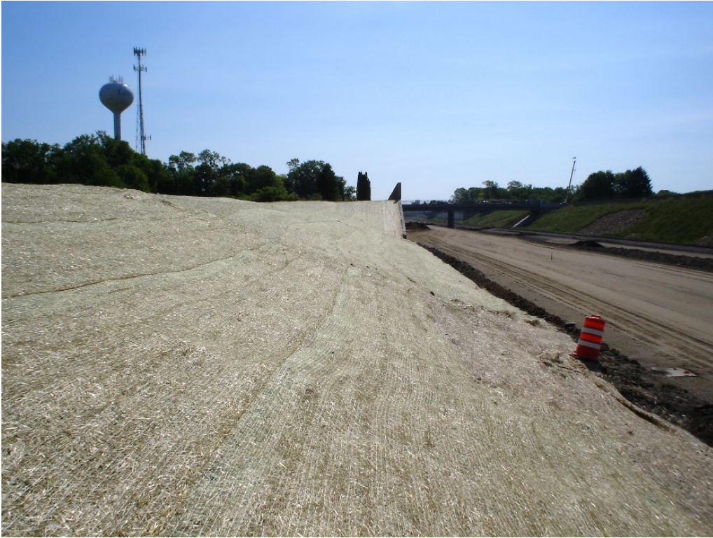
This slope appears to have no vegetative cover, as well as adjacent ongoing construction, and would not be acceptable.
