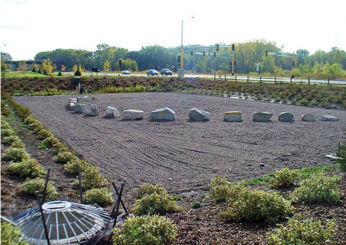
This sand filter system is intended to have a non-vegetated surface. Photo courtesy of Ramsey-Washington Metro Watershed District .
