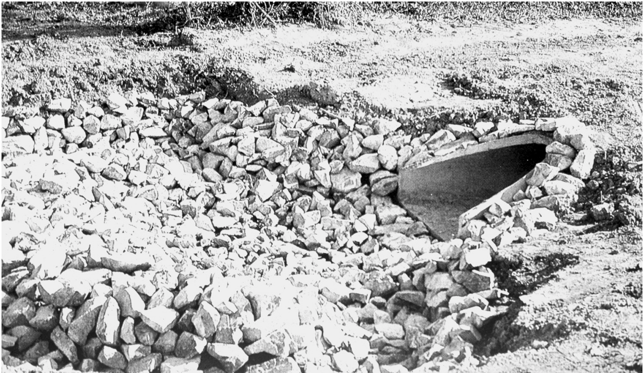
Figure 4.53-2 Outlet protection using riprap
